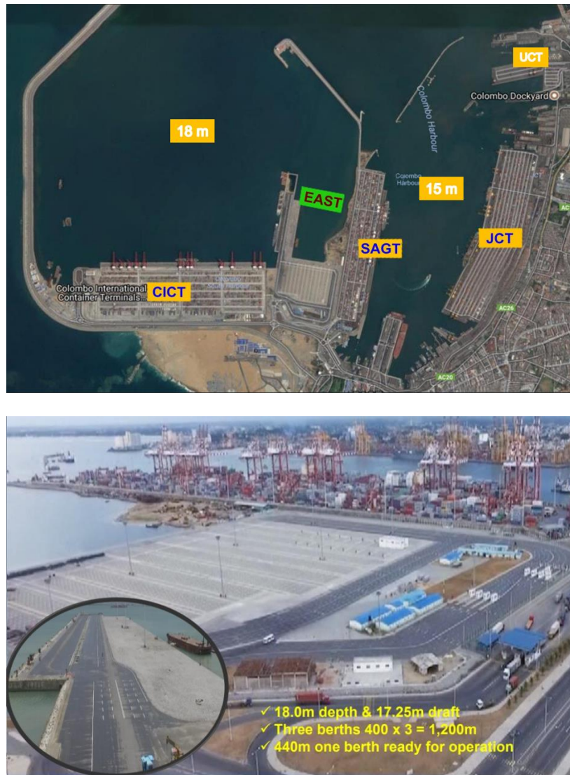
Figure 2: Partly Completed East Container Terminal by SLPA
